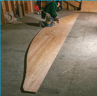
Storyboarding. After tracing the contour from where the trim will be installed, the plywood template is cut and then secured to the subfloor for further templating.
