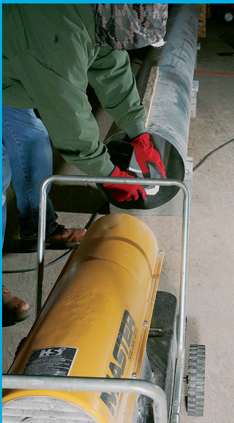
Load when ready. The oven is preheated for about five minutes before loading the trim. Depending on the outside temperature, it can take 30 minutes to an hour to get the trim up to a bendable temperature.
