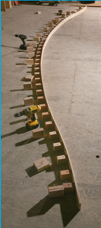
Plenty of room. After the surrounding area is cleared, drivers are set within reach, and 2x blocks loaded with screws are staged for bracing the crown once it's in place.
